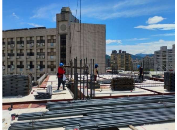
7F 樑筋吊掛
